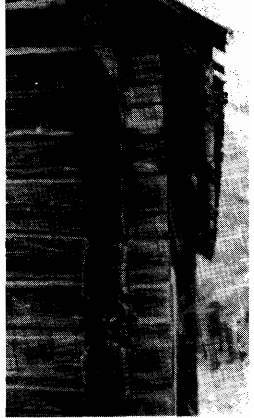
Lock joint cornering
