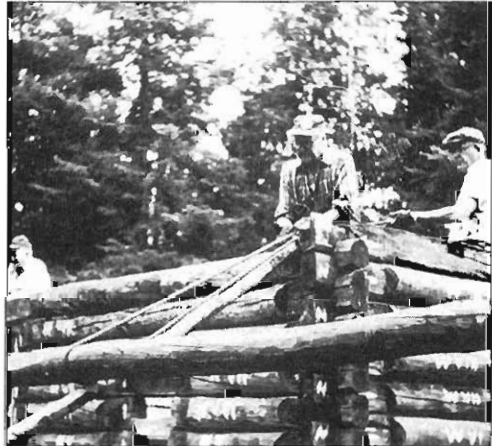
All the timbers were carefully marked at each end, and the weathered tamarack logs were pulled into their respective places. Note the typical Finnish corner notches.
