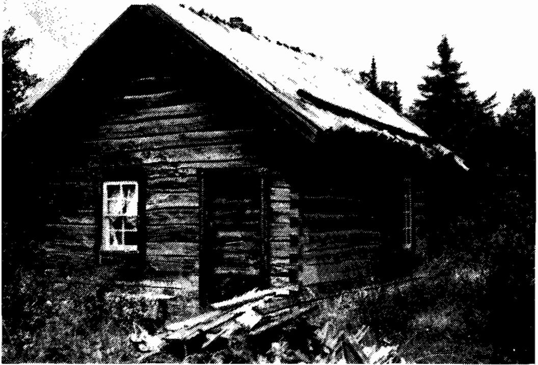
Finnish house in Thunder Bay, note pole roof
