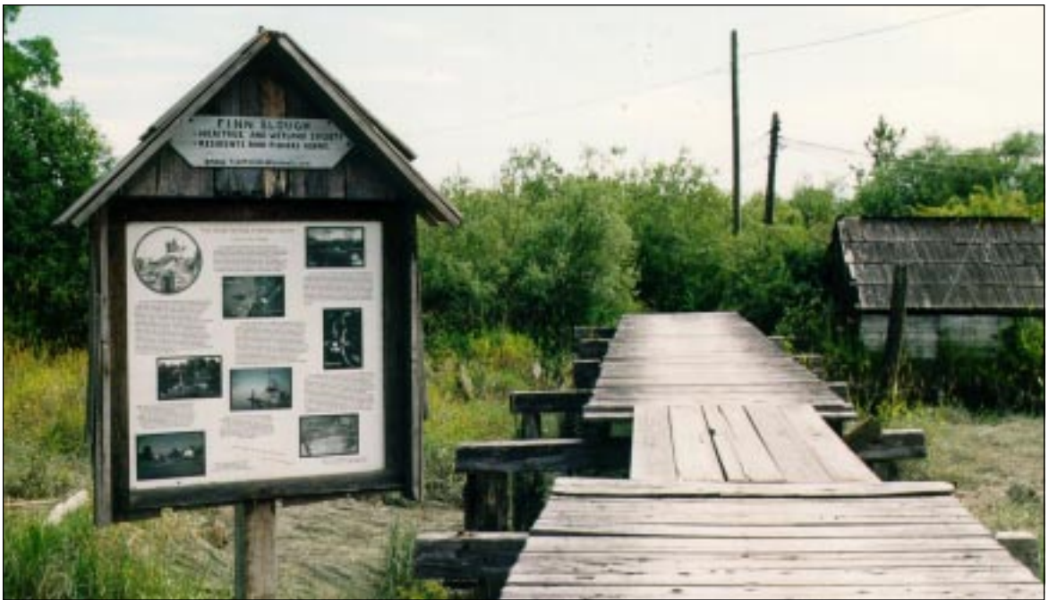
The only “draw bridge” in Richmond. When a new bridge was needed between Gilmour Island and the North bank of Finn Slough, the Anglo British Fishing Company donated all the required lumber. The fishermen gave their skills and labour voluntarily for the common cause. When a fisherman wants to take his boat through the “draw bridge” he simply draws four planks out, takes his boat through, and replaces the planks. The bridge was so well constructed in the 1940's that it is still in use today. – Photo: Jouni Korkiasaari.
